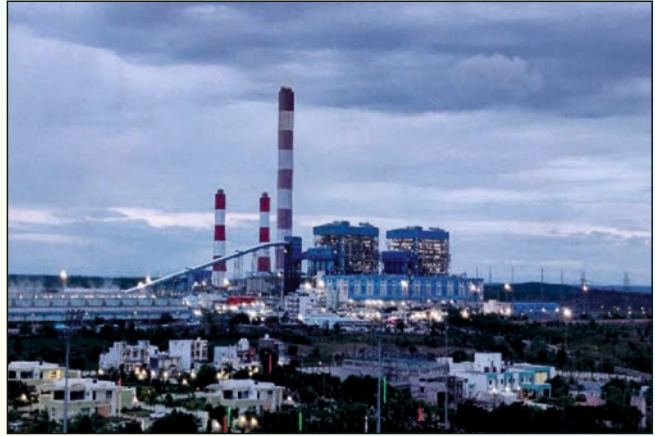
View of Plant
